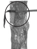
FIGURE 16 TREE BRACE IN- STALLED
